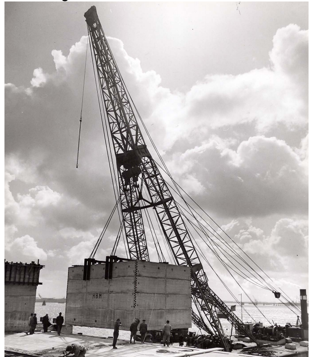
Caissons Waalhaven Rotterdam 1953
