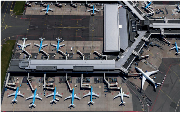
D-pier Schiphol; in 2014 vernieuwd
